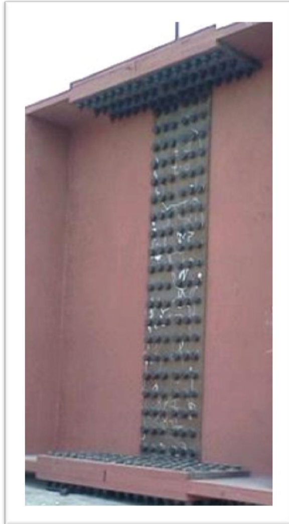
Typical splice joint with HSFG bolting assembly
