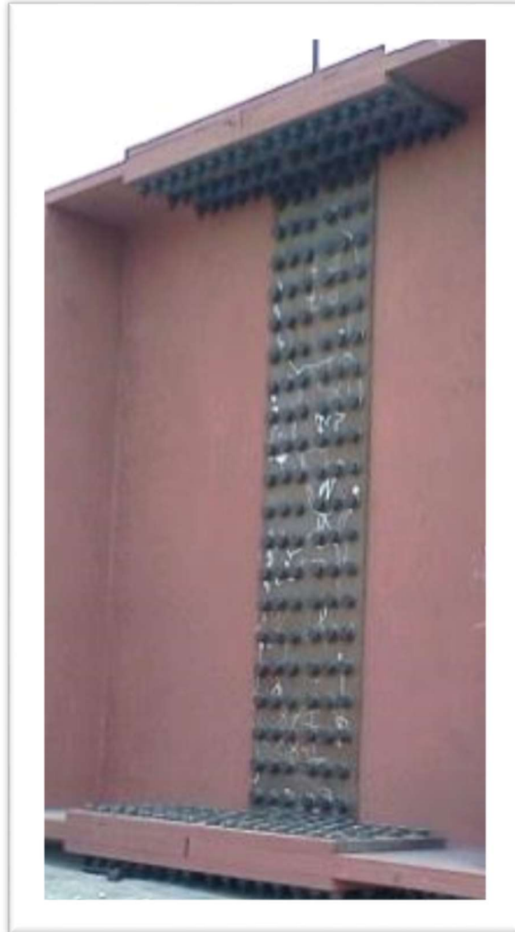
Typical splice joint with HSFG bolting assembly
